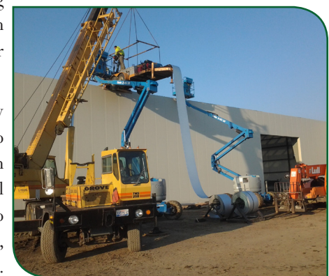
Roof going on May 13, 2016
