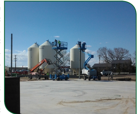
Construction Started April 13, 2016
