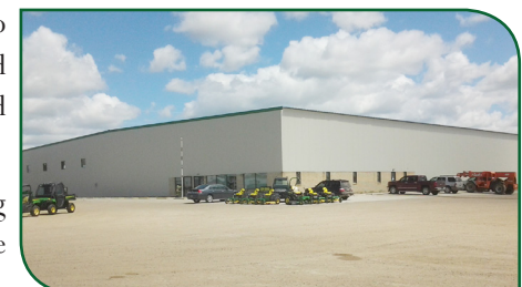
Completed Sheeting on June 1, 2016
