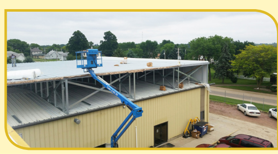
New Roof on Existing Building → 6-12-15
