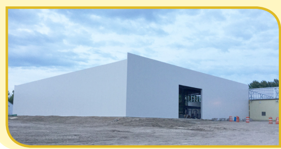
← New Shop Addition 5-29-15
