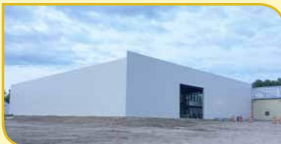
← New Shop Addition 5-29-15
