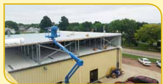
New Roof on Existing Building 6-12-15 →
